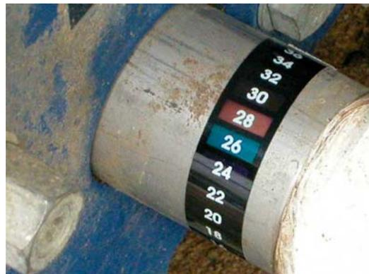
A strip thermometer attached to the milk outlet pipe.
