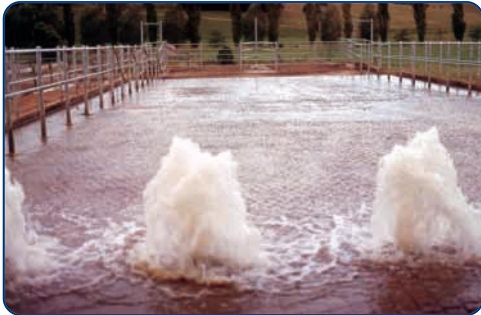
Figure 6.8: Flood wash system with sub surface riser.
