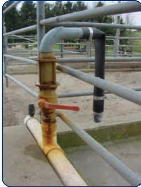
Figure 6.5: Hydrants with an industrial swivel are safer to use.
