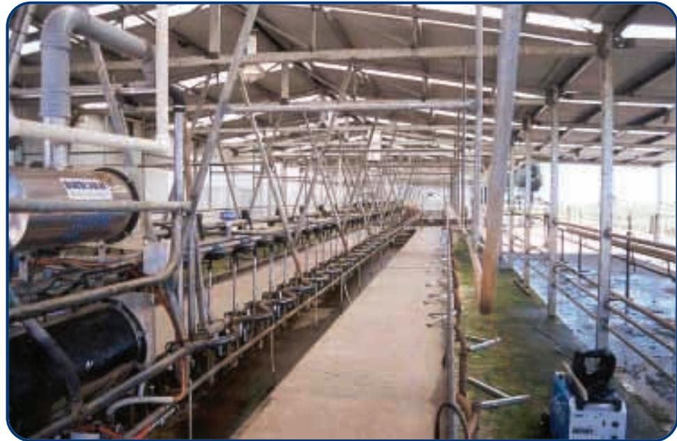
Figure 4.10: Good open dairy design with straight in, straight out cow movement through the dairy.
