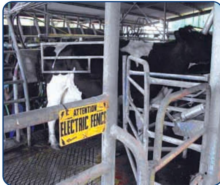
Figure 4.13: Electric fence units and wires that contact dairy pipework are a common source of stray voltage.
