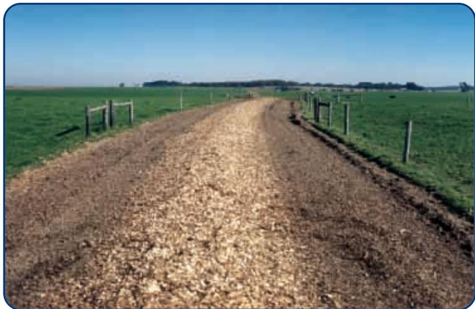
Figure 3.6: Wood chips covering the laneway surface.
