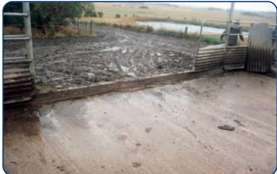
Figure 3.11: Kerb at the yard track junction prevents the wash water from flowing onto the track.
